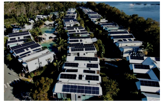
Noosa Lakes Resort – an example of a strata complex taking advantage of the financial benefits from solar
