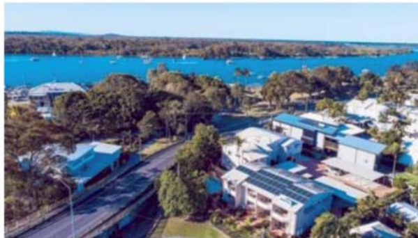
Noosa Sun Motel showing solar panels.
