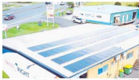
Solar-powered Haymes Paint Shop on Eumundi Road.
